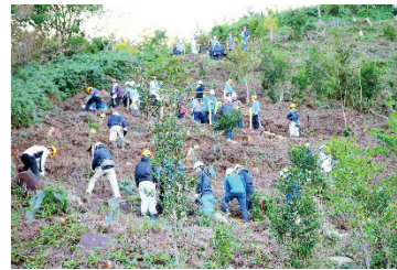
Reforestation work on slopes
