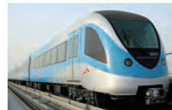
Dubai Metro (Rail Transit System)
