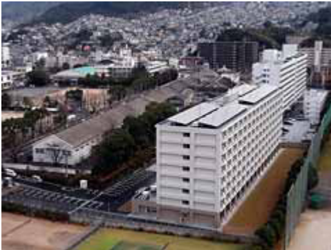
Solar cell panels introduced at MHI single employee dormitories
