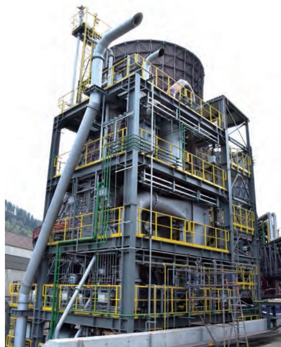
Figure 21 Hydrogen-based fine ore direct reduction (HYFOR) pilot plant
