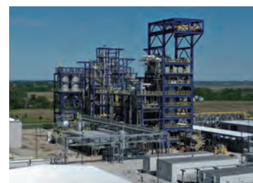
Figure 19 Production plant in operation in Nebraska, U.S., with 14,000 tons/year capacity
